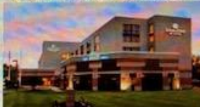
DoubleTree, Hilton Hotel Bradley Airport
